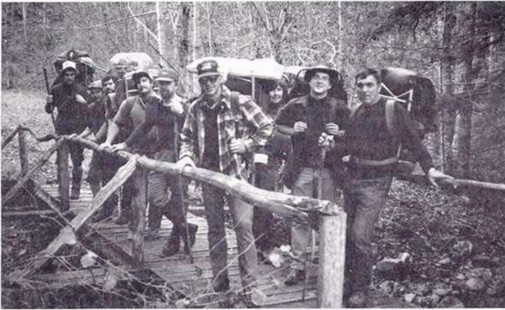
On Camp Carson Bridge.
